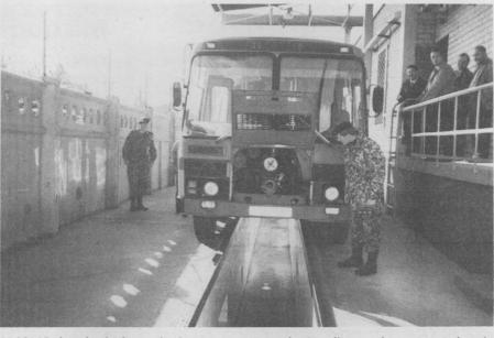
AMONG the physical security improvements at the Ignalina nuclear power plant in Lithuania is this inspection trench similar to a 10-minute oil change bay. From this pit, guards can inspect the undercarriages of vehicles entering or leaving the plant.
